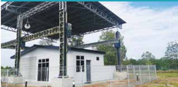
The complete building of a 3D printed sample house
