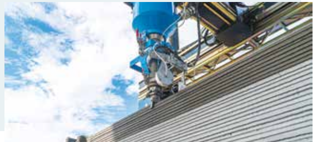
3D Modular Construction Printer from COBOD, Denmark
