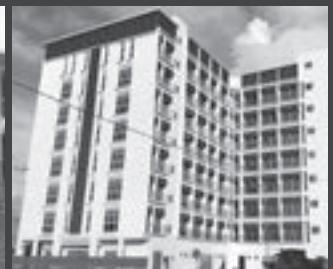
8 Stories Apartment, Bintulu -Supply of IBS precast hollow core slabs and precast beams
