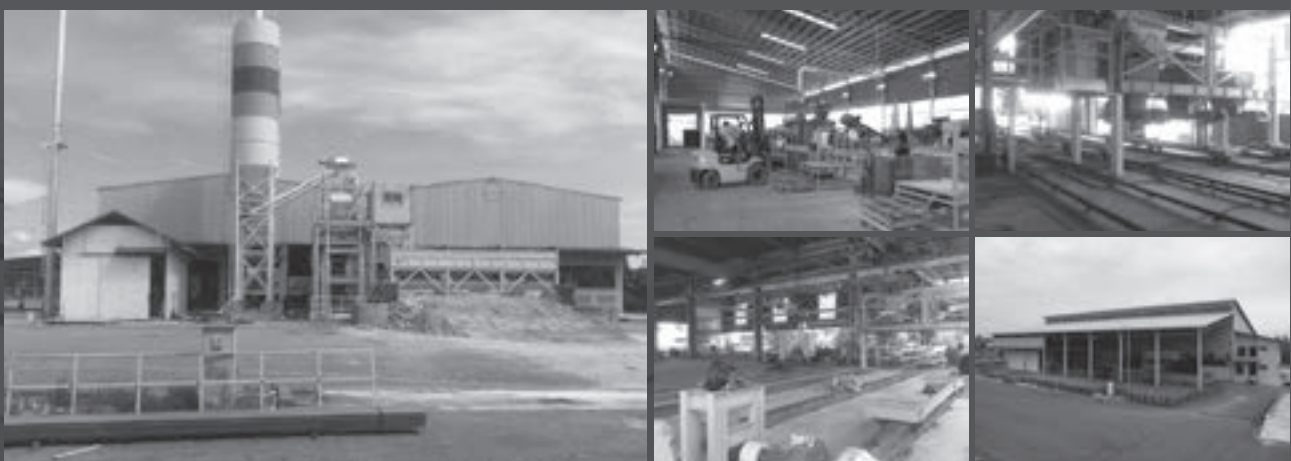
Roofing Tiles, Light Weight Blocks and Spun Pile Factory, Demak Laut Industrial Park, Kuching
