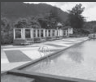
The Cove, Santubong Kuching -Supply of IBS precast hollow core slabs and precast beams
