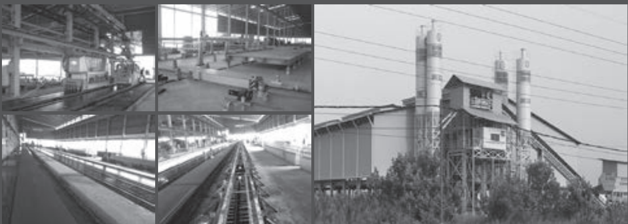
IBS Factory, Demak Laut Industrial Park, Kuching
