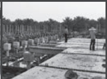
KUB Mill at Mukah - Supply of IBS hollow core slabs and square piles
