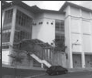
Central Teaching Faculty for UNIMAS - Supply of IBS components and spun piles
