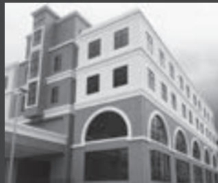
Sego Centre, 4 Storey Office Building, Petra Jaya - Supply of precast column, precast beams and IBS hollow core slabs
