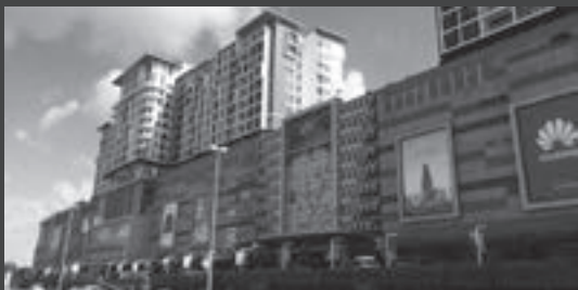
Vivacity Project - an integrated mixed development comprising a retail podium and 4 blocks of service apartments at Jalan Wan Alwi, Kuching - Supply of IBS components and spun piles
