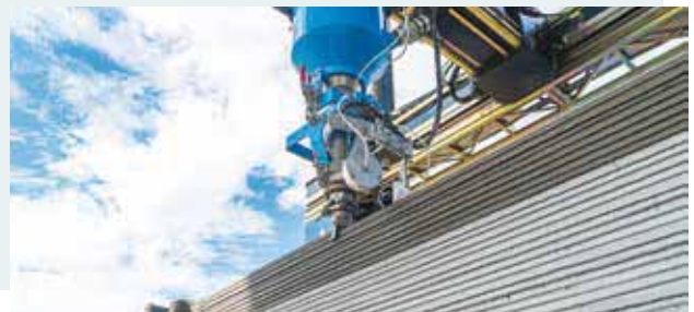
3D Modular Construction Printer from COBOD, Denmark
