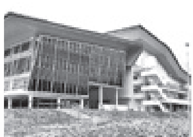
Pusat Islam for UNIMAS - Supply of IBS components and Spun piles
