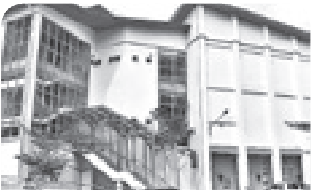
Central Teaching Faculty for UNIMAS - Supply of IBS components and Spun piles
