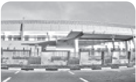
Proposed Klinik Kesihatan Jenis 3XP on Lot 3081 & 3082, Malaysia - Supply of IBS components
