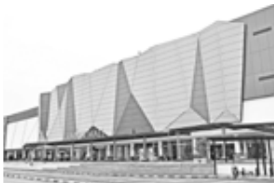
The Summer Mall - Supply of IBS components and square piles
