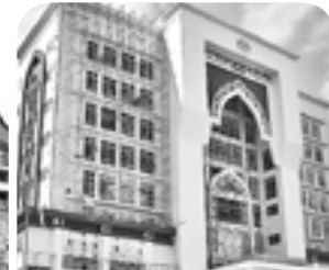
Royal Custom Malaysia Sarawak Headquarter - Supply of IBS components
