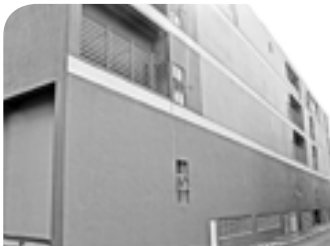
Three Storey Commercial Complex at Jalan Wan Alwi - Supply of IBS components and square piles
