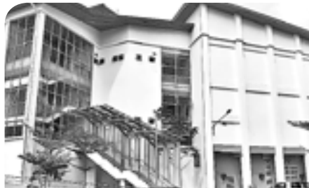
Central Teaching Faculty for UNIMAS - Supply of IBS components and spun piles
