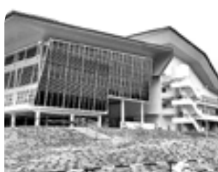
Pusat Islam for UNIMAS - Supply of IBS components and spun piles
