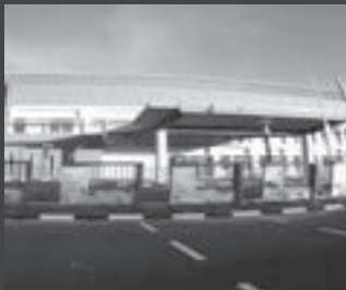
Klinik Kesihatan Jenis 3XP on Lot 3081 & 3082, Malaysia - Supply of IBS components
