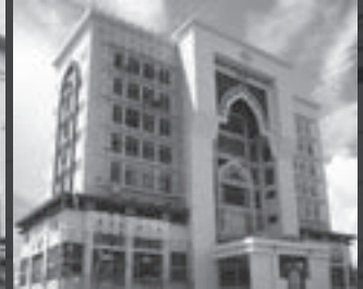
Royal Customs Malaysia Sarawak Headquarter - Supply of IBS components
