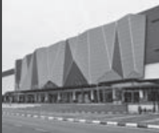
The Summer Mall - Supply of IBS components and square piles
