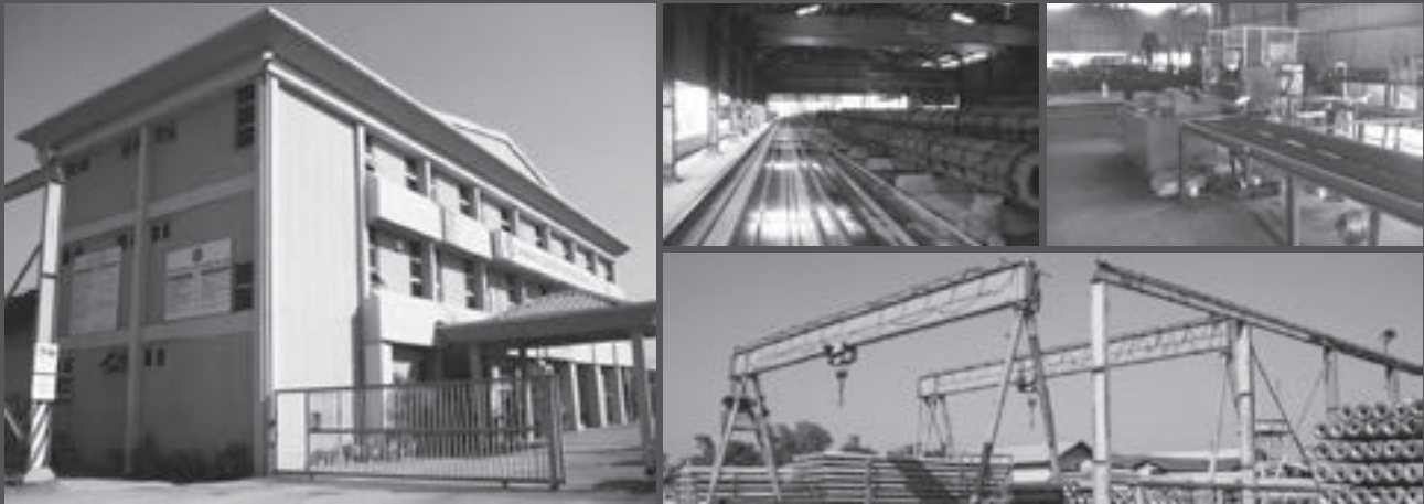
Main Factory, Pending Industrial Estate, Kuching
