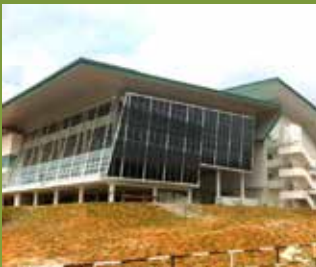
Pusat Islam for UNIMAS - Supply of IBS components and spun piles
