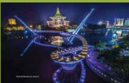
Darul Hana Bridge, Kuching -Supply of precast plank
