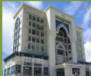
Royal Customs Malaysia Sarawak Headquarter - Supply of IBS components
