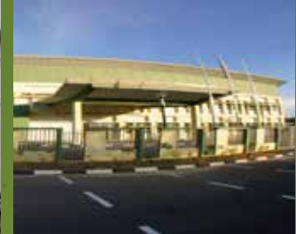
Klinik Kesihatan Jenis 3XP on Lot 3081 & 3082, Malaysia - Supply of IBS components
