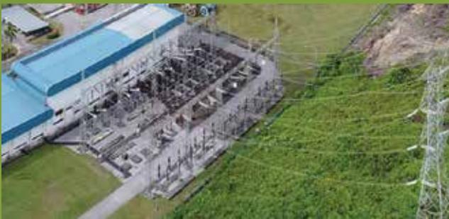
Power Utilities Sub Station - Supply of foundation piles
