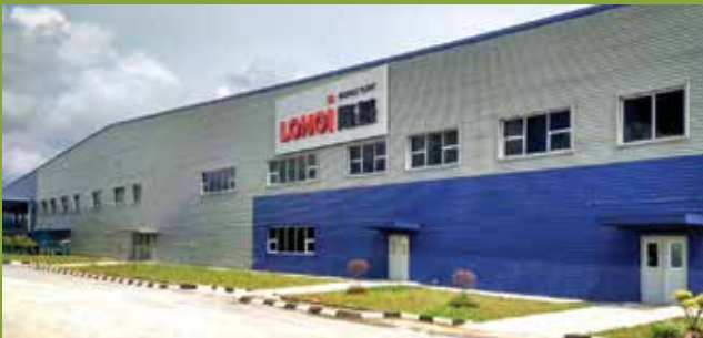
Solar Panel Factory in Samajaya Industrial Park Kuching - Supply of foundation piles
