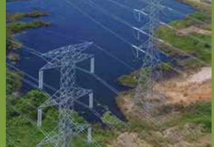
Sarawak Power Transmission line project - Supply of foundation piles
