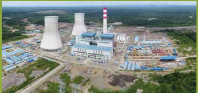
Mukah Coal Power Plant - Supply of foundation piles
