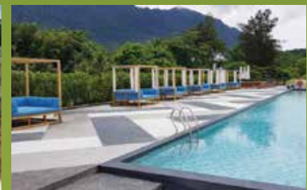
The Cove, Santubong, Kuching - Supply of IBS precast hollow core slabs and precast beams
